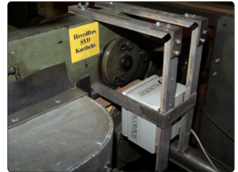
Scorpion Laser Profile Measurement System installation
