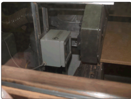
Junction box installed
